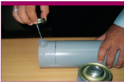
Apply equal quantity of solvent cement to the spigot (not to exceed the marked line) & the socket
