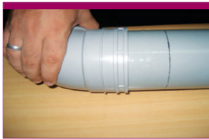
Push the spigot & the socket together while the solvent cement is wet & hold for at least for 30 seconds to allow the dryness of the solvent cement
