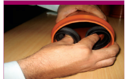
Insert the rubber ring as shown in the socket of the pipe
