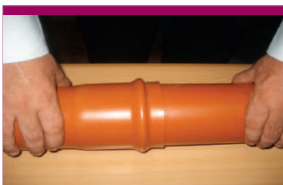
Push firmly the socket & the spigot to each other until the marked socket depth line is covered
