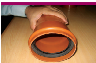
Make sure that the rubber ring is firmly in the socket with no edges out of the ring groove
