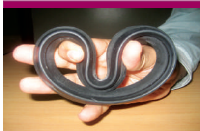
Fold the rubber ring as shown preparing it to the socket
