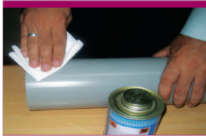
Remove all dust made by the Chamfering & any trace of grease inside & outside the edge of the pipe with dry & clean cloth
