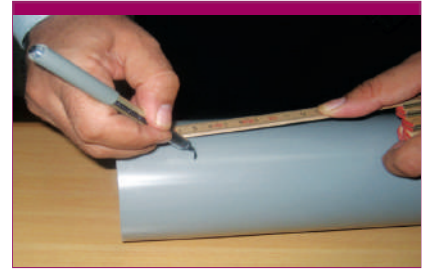
mark the spigot with the same depth of the socket prior to applying the solvent cement
