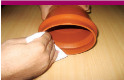
Clean the socket from any dirt or grease specially the inside the ring groove
