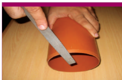
Chamfer the spigot side of the pipe before sliding it to the rubber socket in the pipe or the fitting
