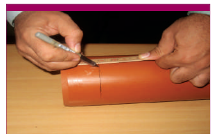
Mark the depth of the socket on the spigot
