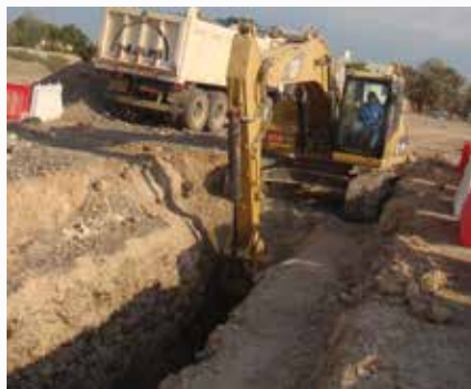
Trenching at Oman
