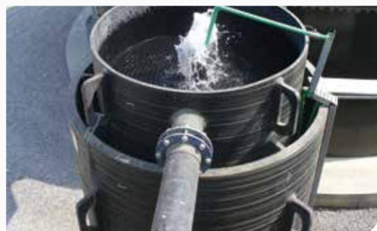
NIC HDPE Corrugated Pipe used as sewerage water bio treatment plant for project in Oman
