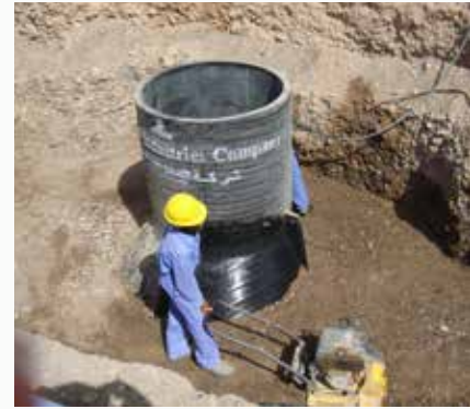
Initial backfill at project in Oman
