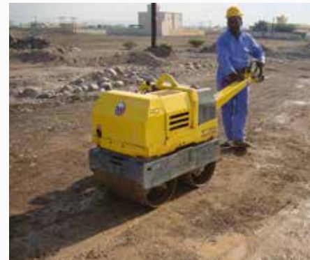
Final Backfill at project in Oman
