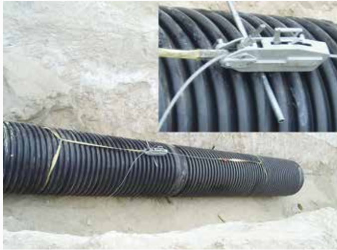
Assembly of pipes at project in Kuwait
