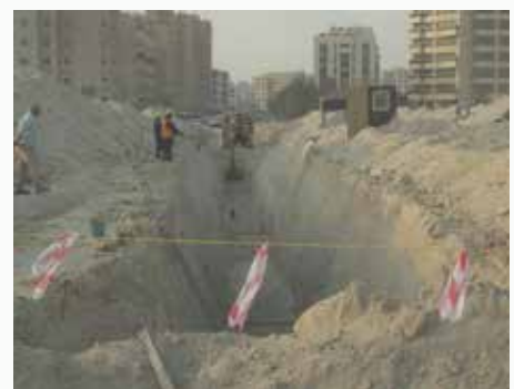
Trenching at Kuwait
