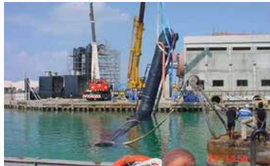
NIC HDPE Corrugated Pipes for sea water intake project in UAE
