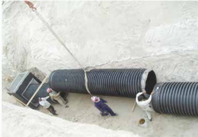
Loading at project in Kuwait
